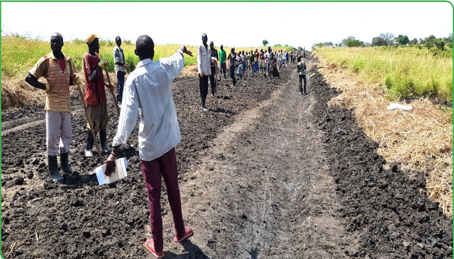
Refugees in Luru Village - Palorinya refugee settlement in Moyo district back filling, slopping & establishing water drainage system undereasn for work
